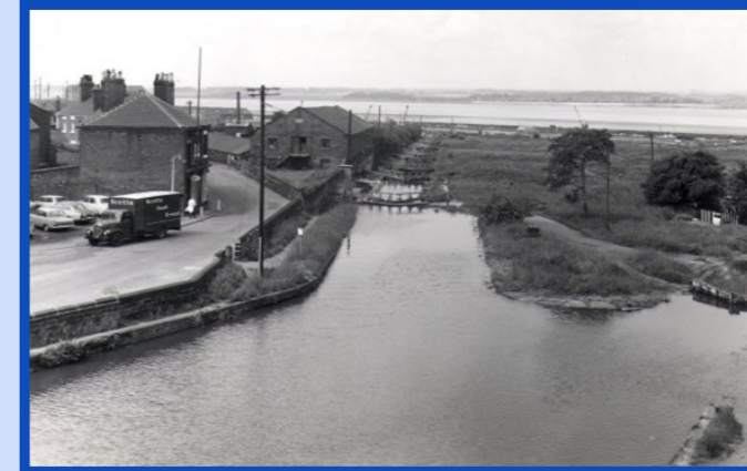
The flight of locks at Runcorn, now demolished
