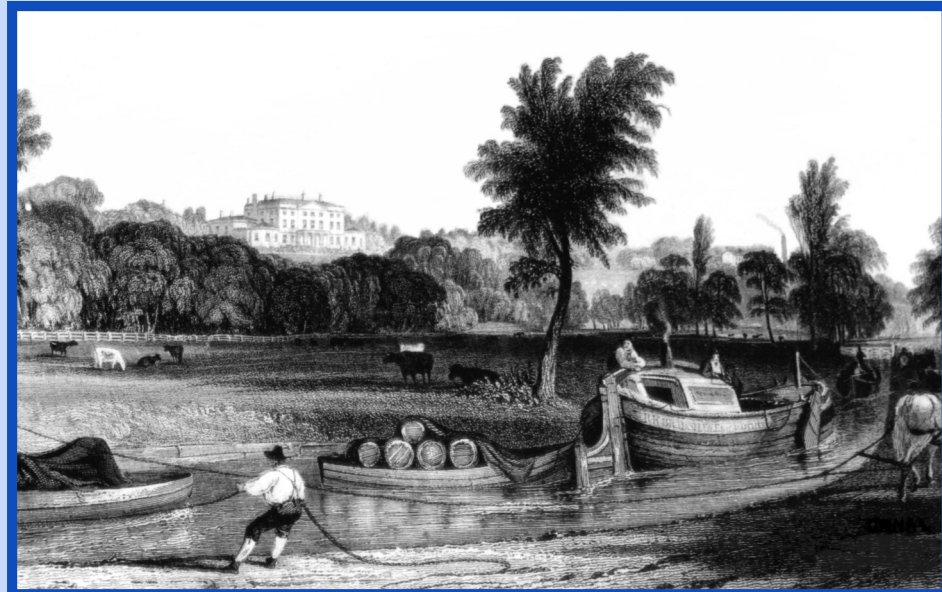
The Brick Hall and Bridgewater Canal
