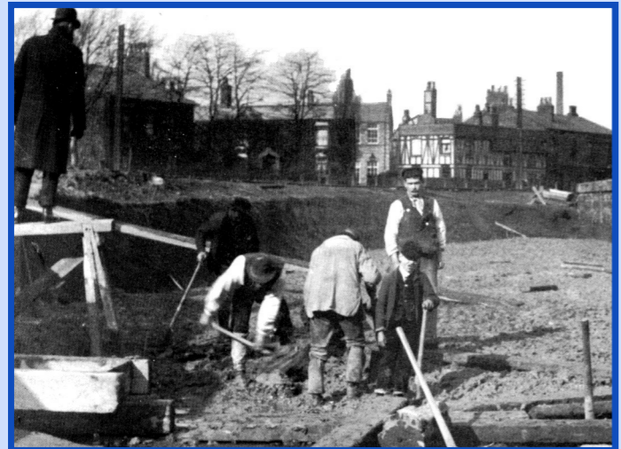
Puddling clay to repair the canal in 1893
