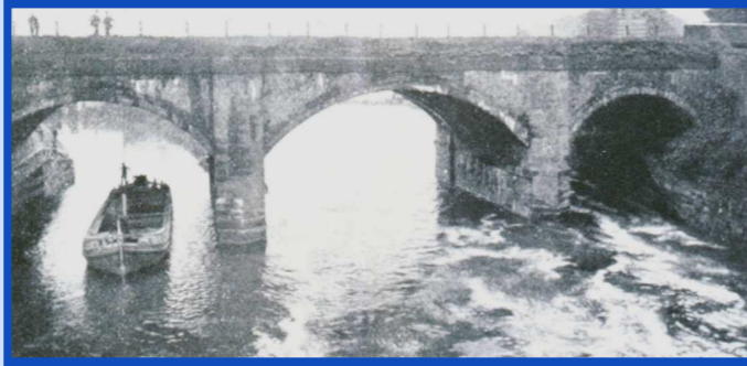
Cutwaters were added to the stonework to minimise erosion
