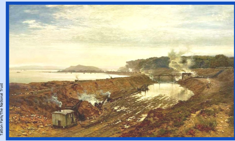
Panorama of the canal entrance at Eastham during construction
